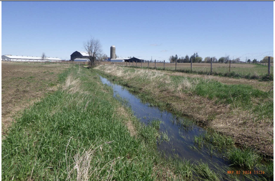
The constructed channel was straightened and flowed between agricultural fields. The channel was entrenched, had a low gradient and lacked canopy cover.
