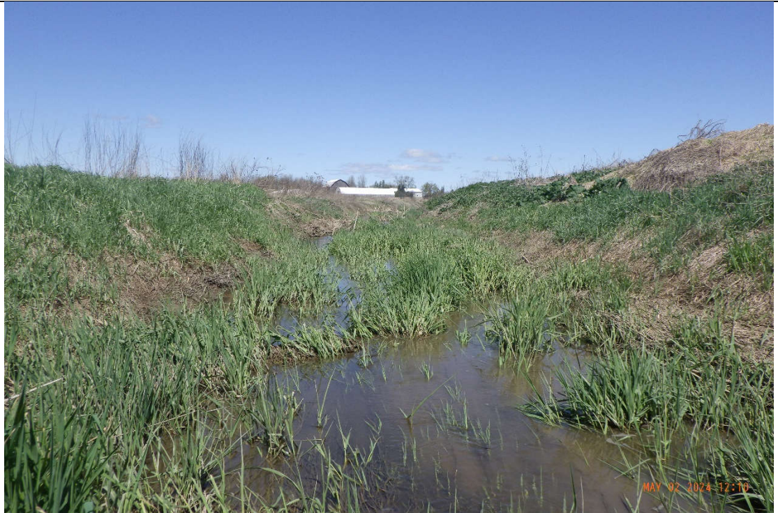
Photo 12 Alloa Drain - Reach AD4, Caledon, Ontario
