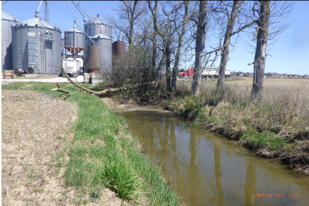
Minimal erosion was observed within the reach, with localized undercutting in the downstream extent. Undercuts of up to 0.30 m were measured.
