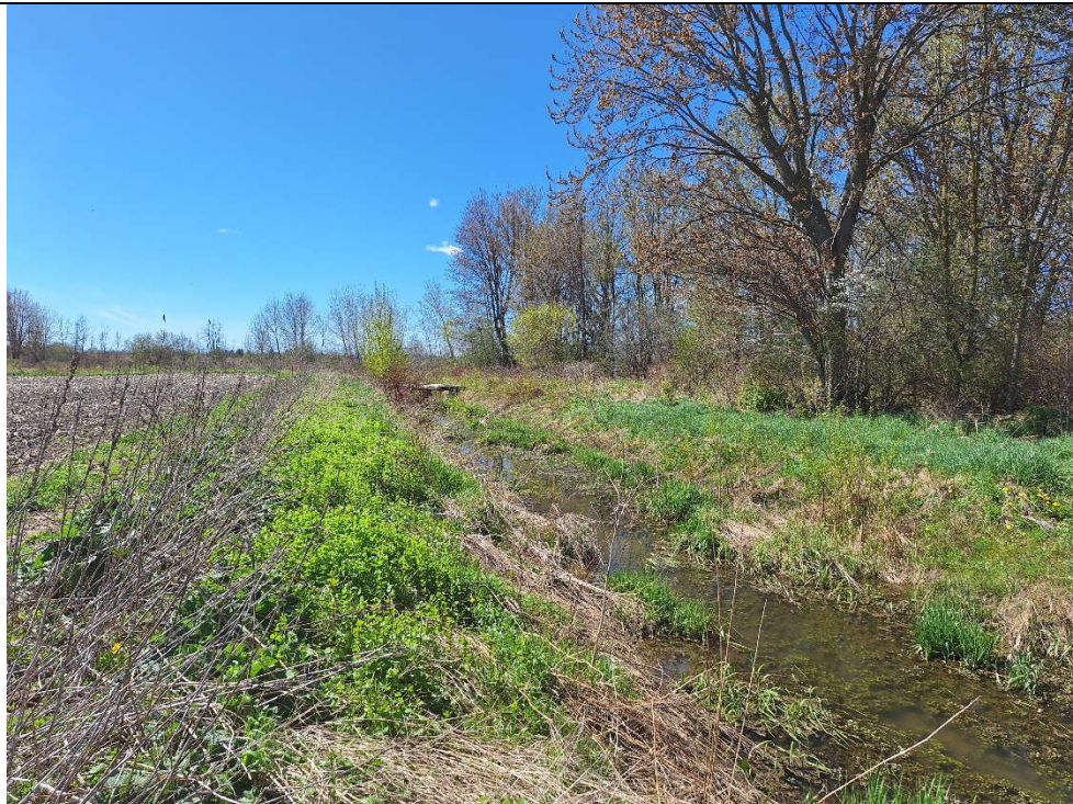
The channel banks were steep and high in the upstream portion of the reach. Lower bank angles were present in the downstream portion of the reach.
