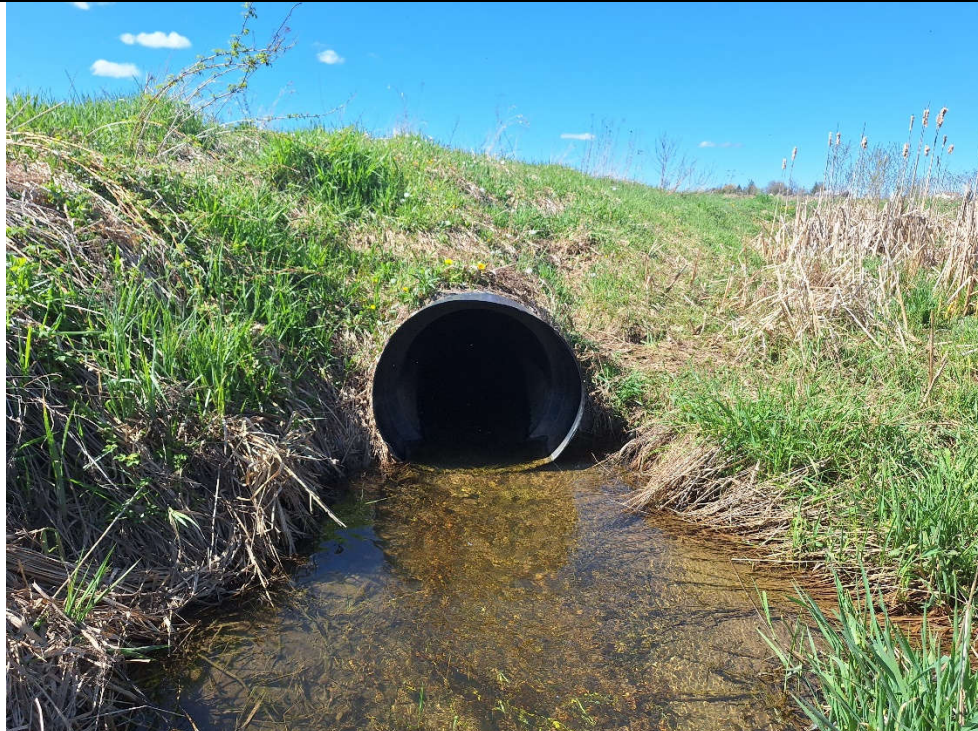
A tile drain (Reach LD5) was observed to discharge at the upstream extent of the reach.
