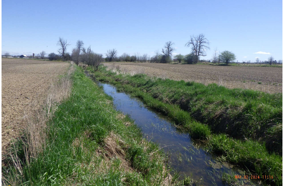
The banks throughout the reach were generally steep, with angles ranging from 60 – 90 degrees.
