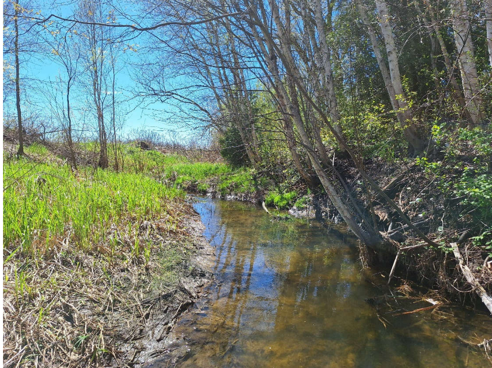
Localized areas of erosion and undercutting were present primarily mid-reach. Undercuts measured up to 0.54 m.
