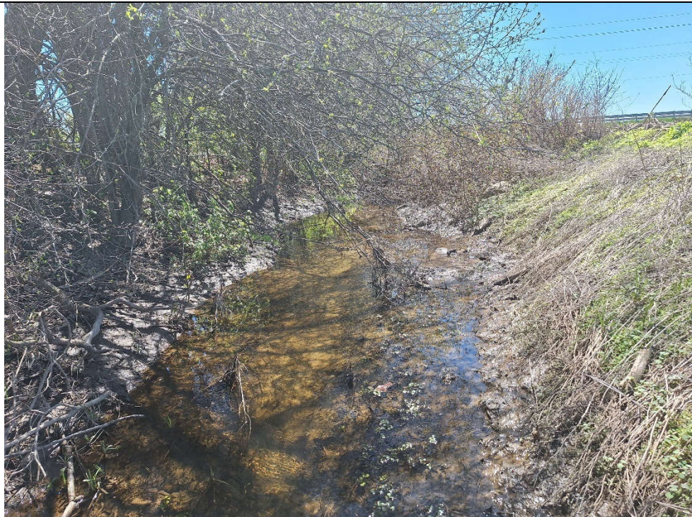
The reach was short and contained a straight channel that had minimal erosion and moderate entrenchment.
