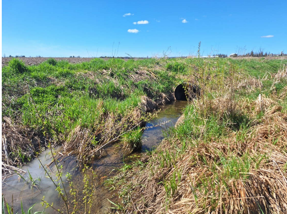
The riparian vegetation primarily consisted of grasses with some trees. The grasses were moderately encroaching into the channel.
