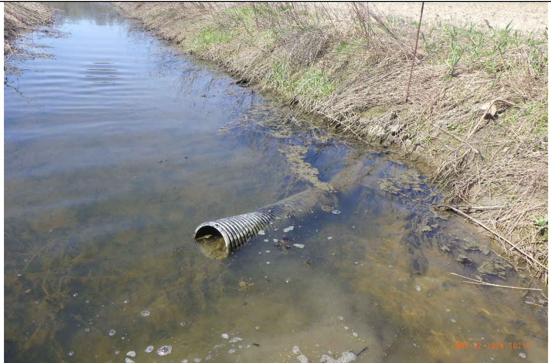
The channel flowed through agricultural fields and multiple tile drains were observed throughout the reach.
