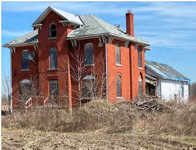
Photograph 11: House likely requiring a future bat exit survey at 12455 Creditview Road (April 9, 2024).
