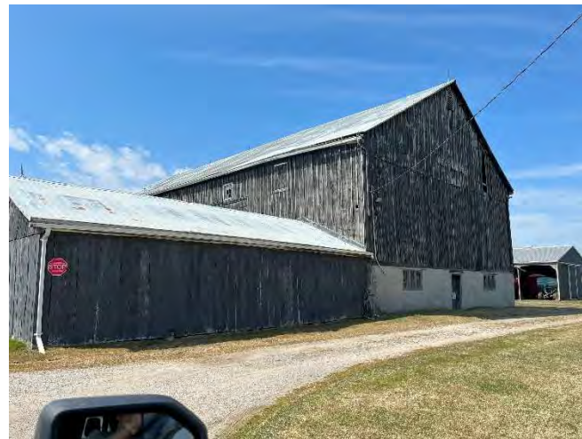
Photograph 12: Barn likely requiring a future bat exit survey at 12300 Mississauga Road (April 9, 2024).
