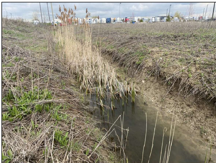
Photo 3. Typical channel cross-section with in-stream vegetation and evidence of channel maintenance.
