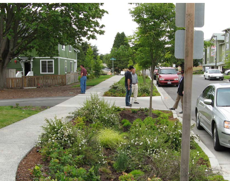
Figure 6.3: Examples of water conservation and management strategies that can be implemented throughout the development
