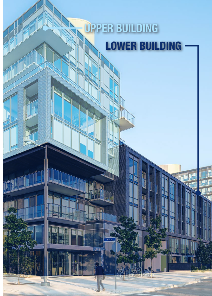
Figure 5.13: Building materials and detailing are used to establish a lower and upper portion of the building
