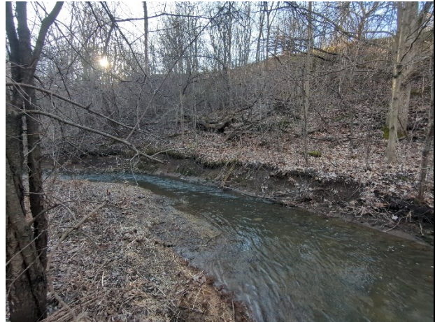
Photo 6 – Valley toe impact in Reach WHT4(3)-2, downstream view.
