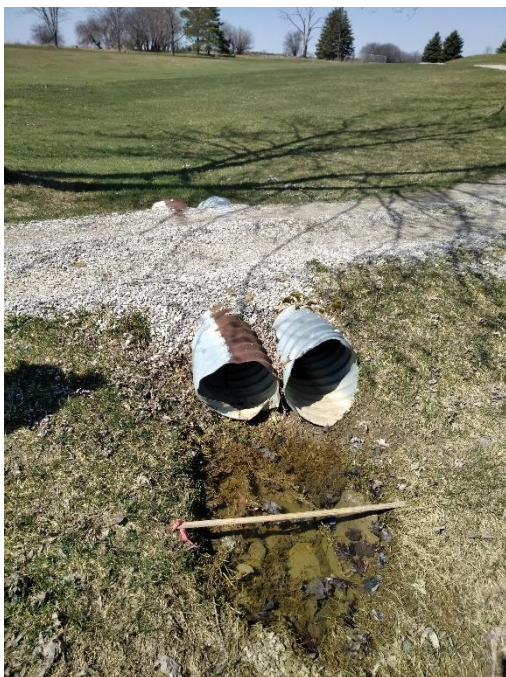
Photograph 14. HDF 4B – Upstream View (April 12, 2023).
