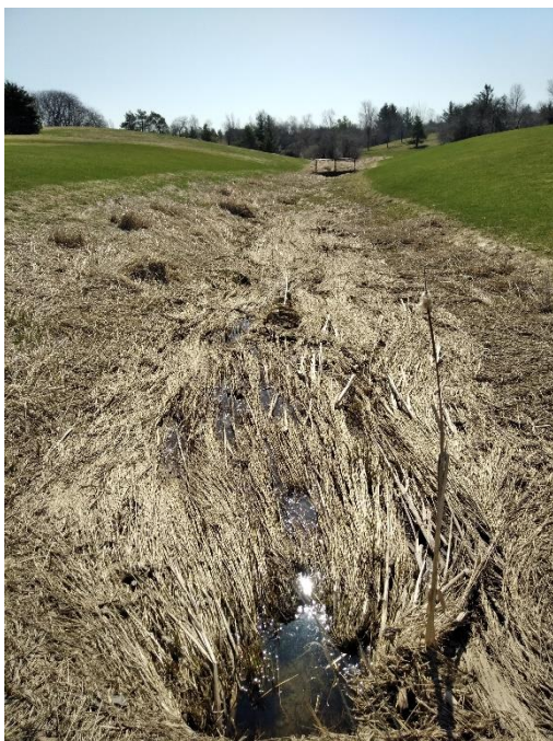
Photograph 10. HDF 3A – Downstream View (April 12, 2023).
