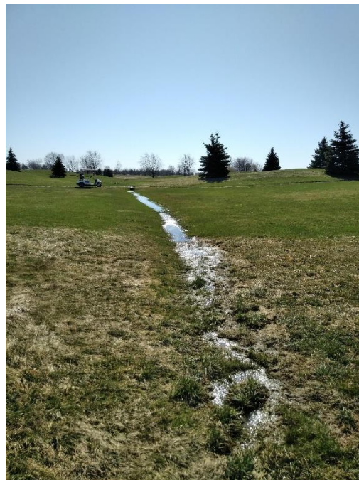
Photograph 9. HDF 2 – Downstream View (April 12, 2023).
