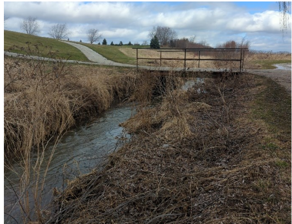
Photo 20 – Reach WHT4(3)2-1 flows under several crossings connecting golf cart pathways.
