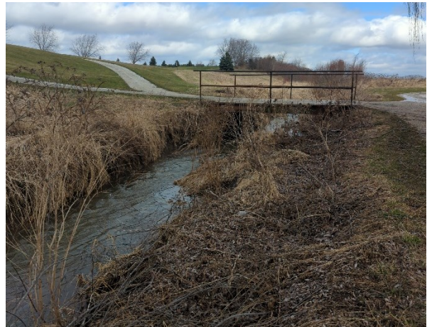
Photo 16 – Reach WHT4(3)2-1 flows under several crossings connecting golf cart pathways.
