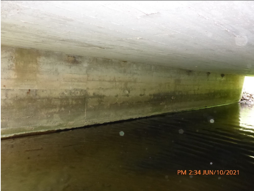
Abutments - Abutment Walls - Typical - West - Photo 19
