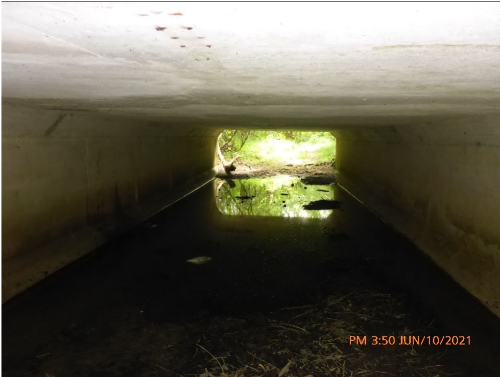
Looking West through Barrel from End - Photo 9
