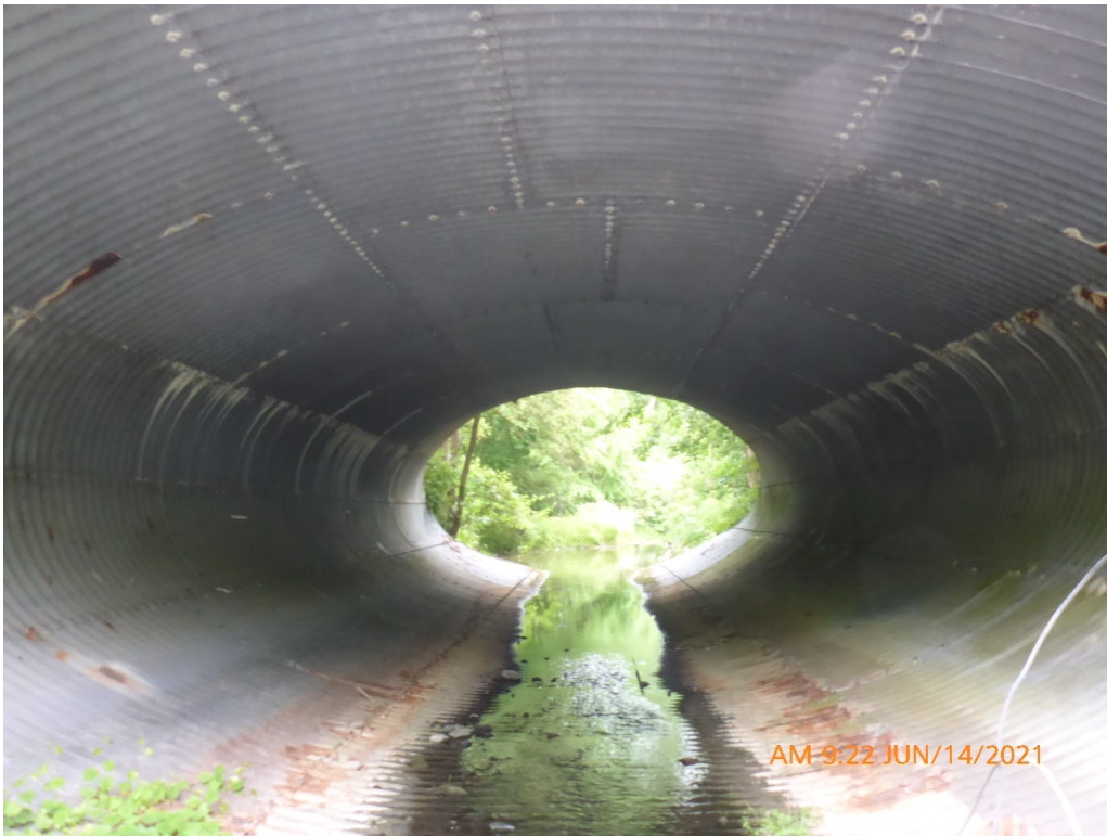
Looking East through Barrel from End - Photo 8
