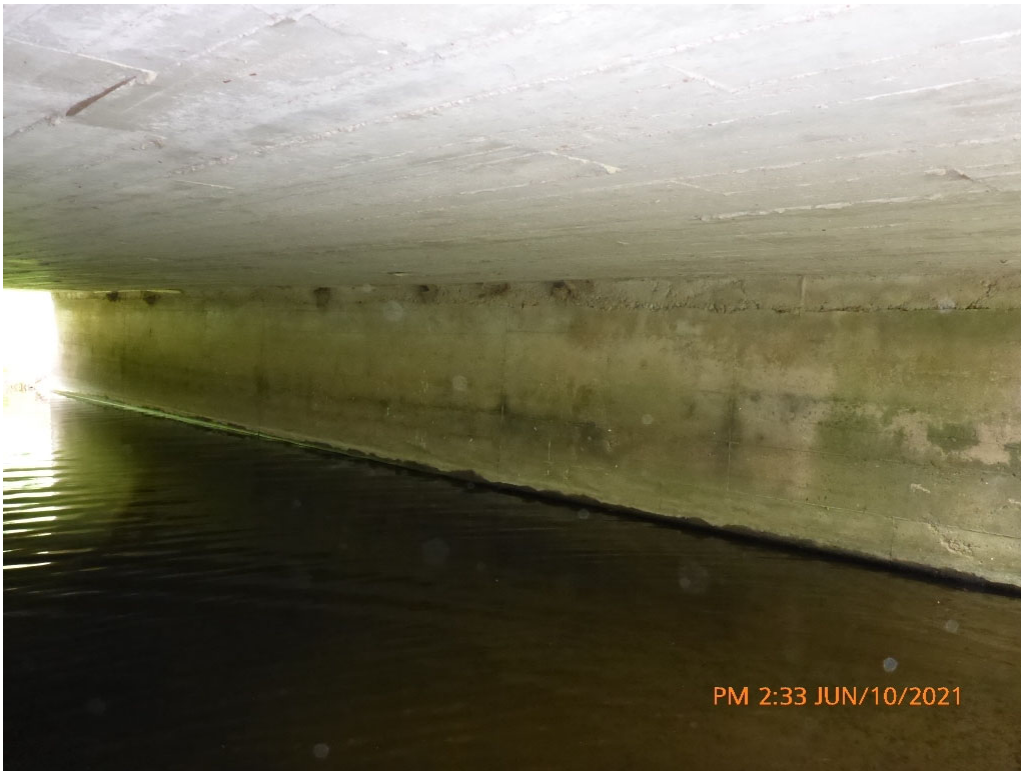
Abutments - Abutment Walls - Typical - East - Photo 18
