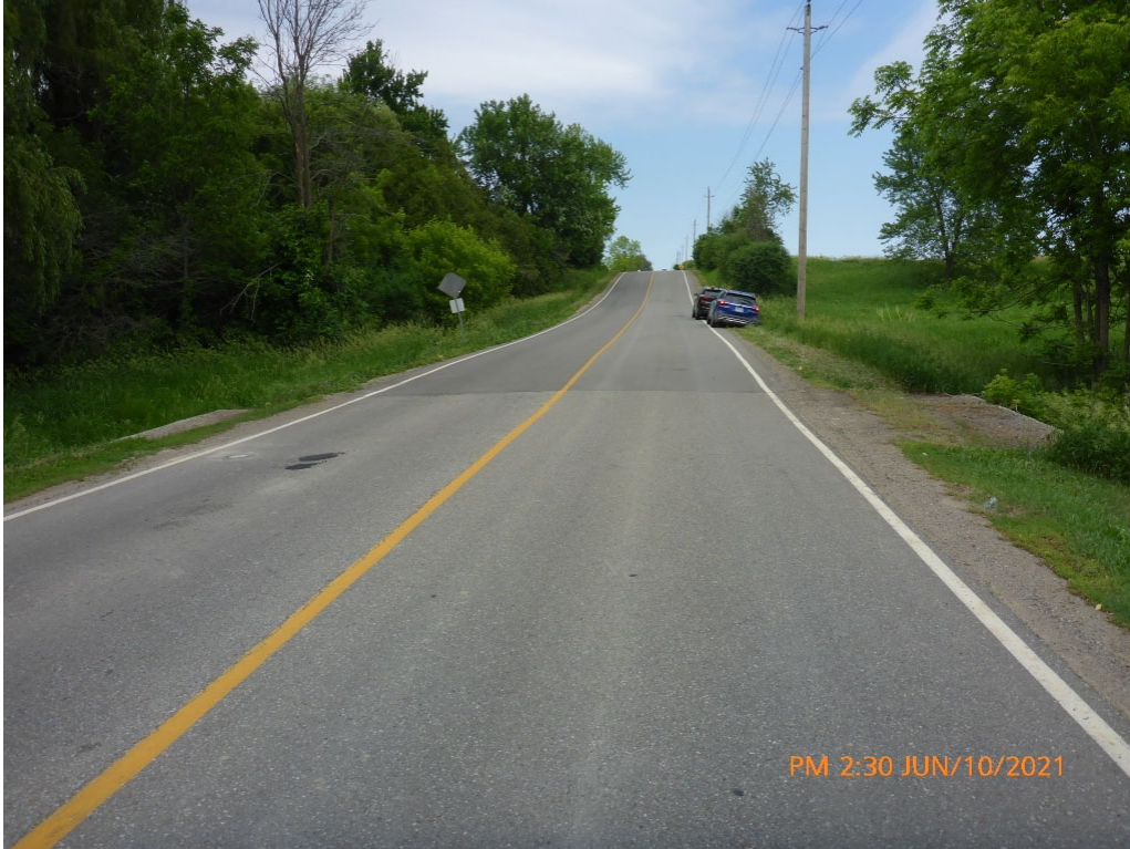
Looking East at Bridge - Photo 1
