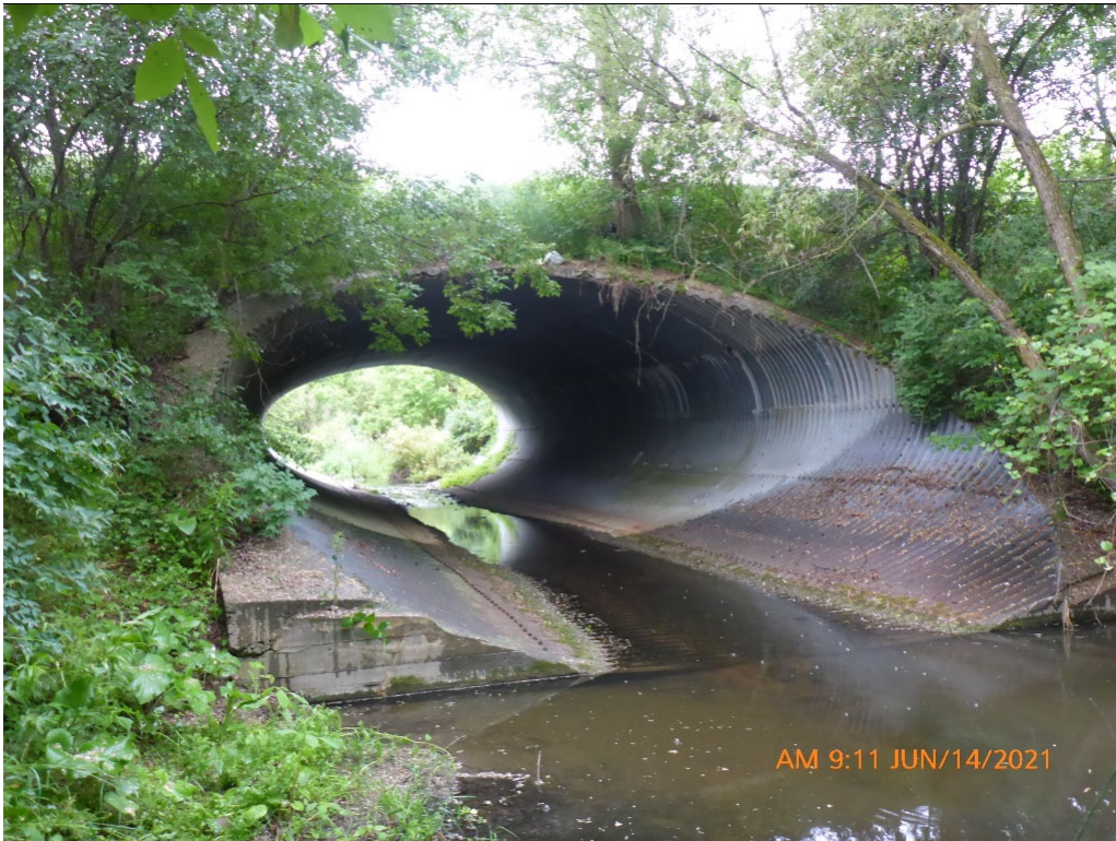
East Elevation - Photo 3
