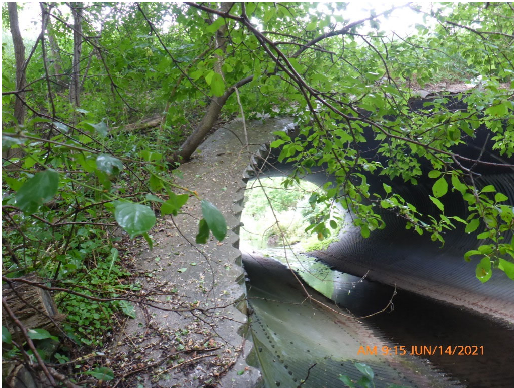
Culverts - Outlet Components - Typical Stiffener - Photo 32
