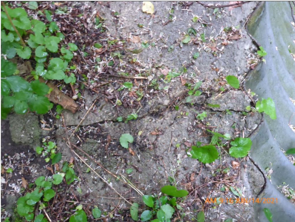
Culverts - Outlet Components - Wide Crack in Stiffener - SE - Photo 33
