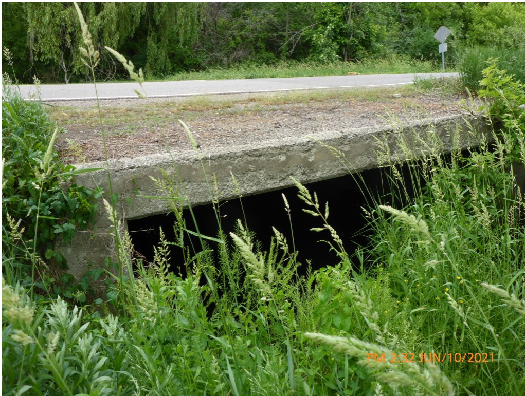
South Elevation - Photo 4
