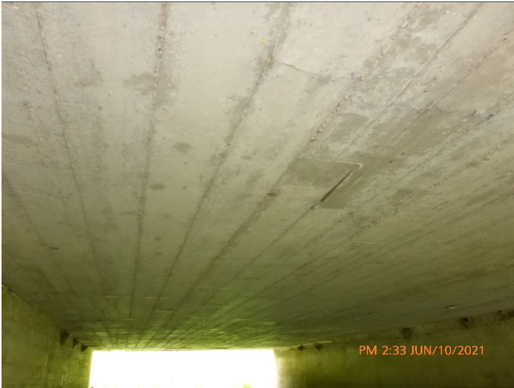
Decks - Soffit - Thick Slab - Typical - Photo 13
