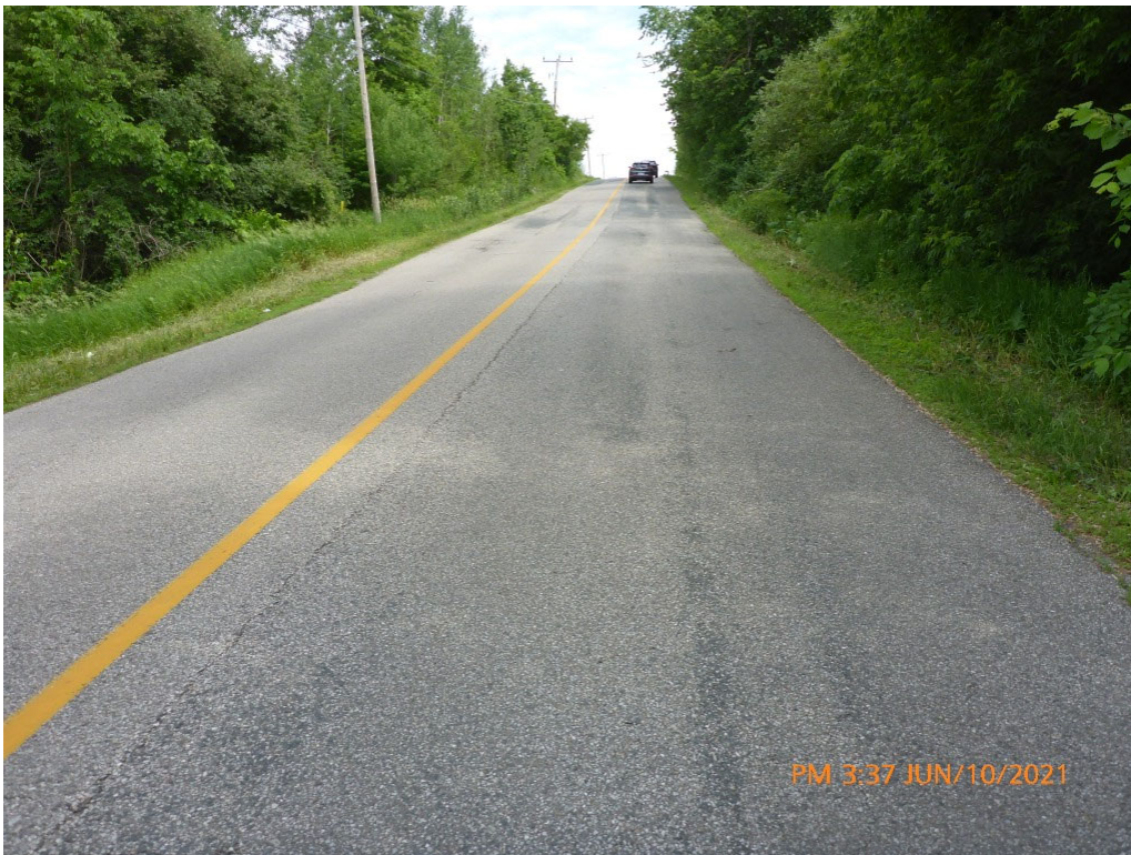
Looking South at Roadway over Culvert - Photo 2
