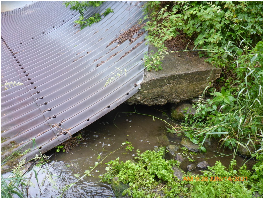
Culverts - Inlet Components - Typical Cut-off Wall - Photo 22
