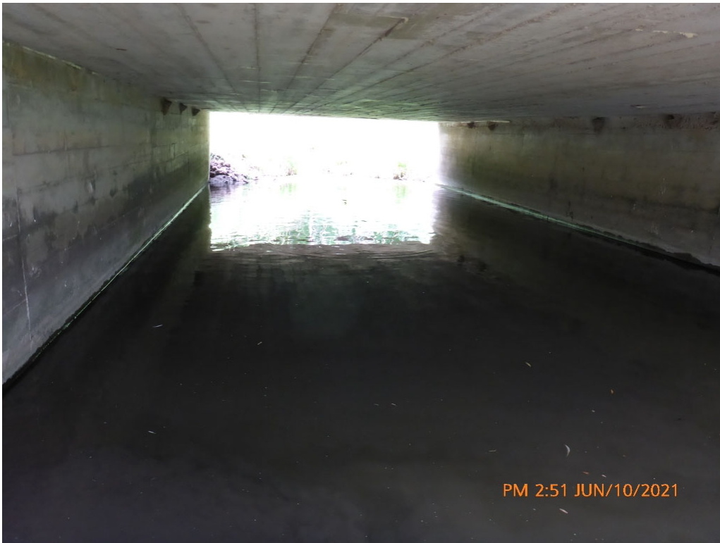
Embankments and Streams - Streams_Waterways - Watercourse Below Bridge - Photo 26
