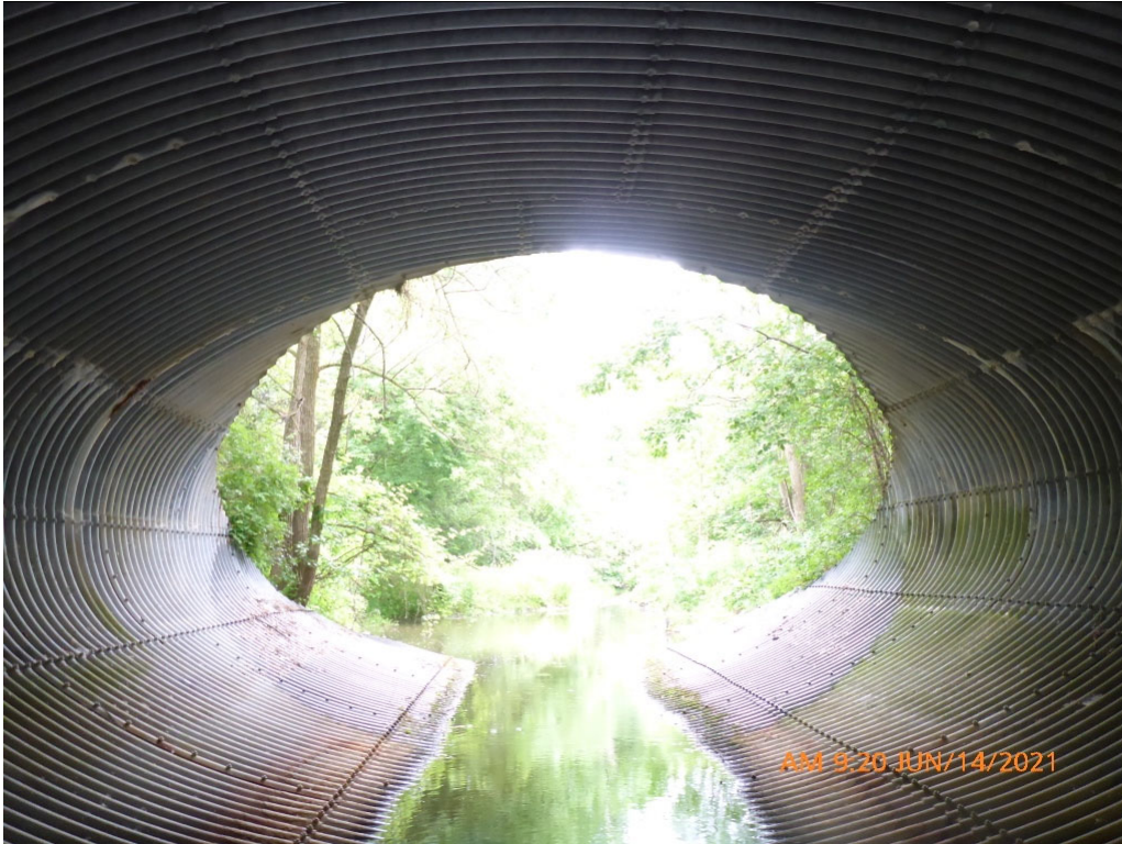
Looking East through Barrel at Midspan - Photo 9
