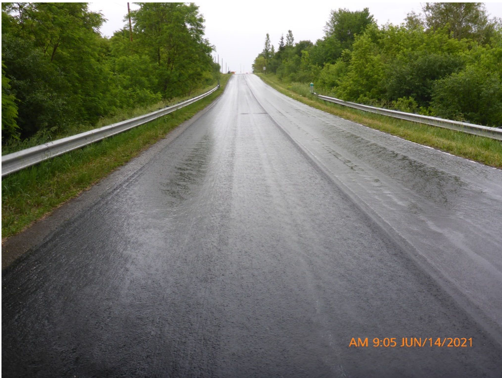
Looking South at Roadway over Culvert - Photo 2
