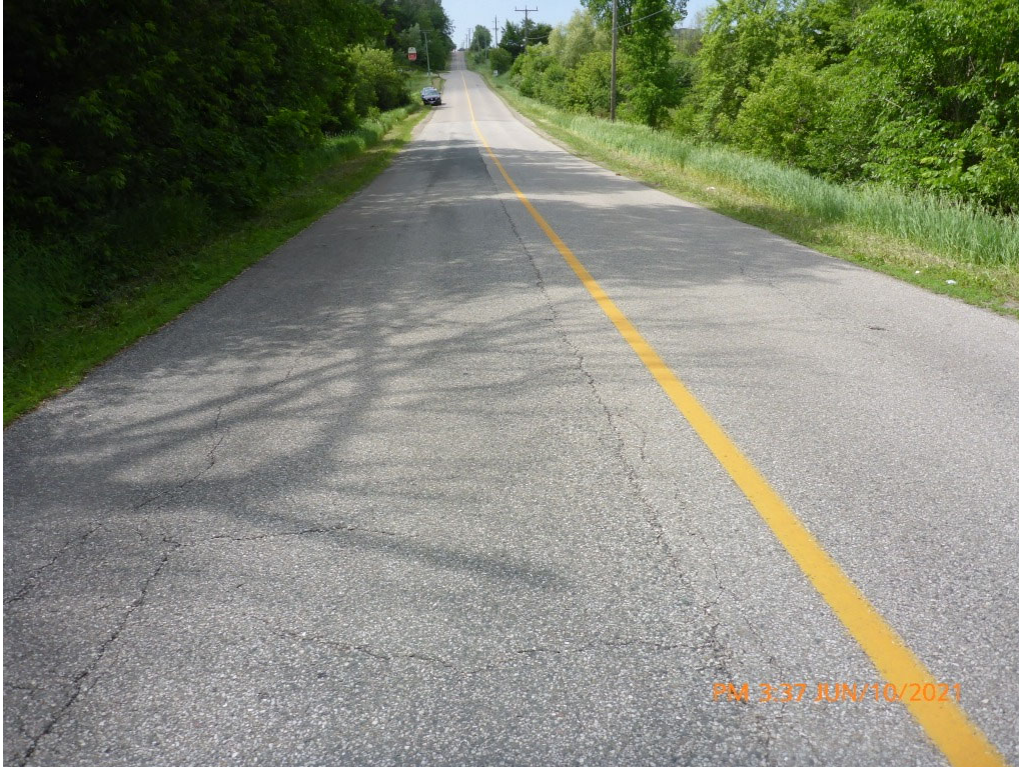
Looking North at Roadway over Culvert - Photo 1
