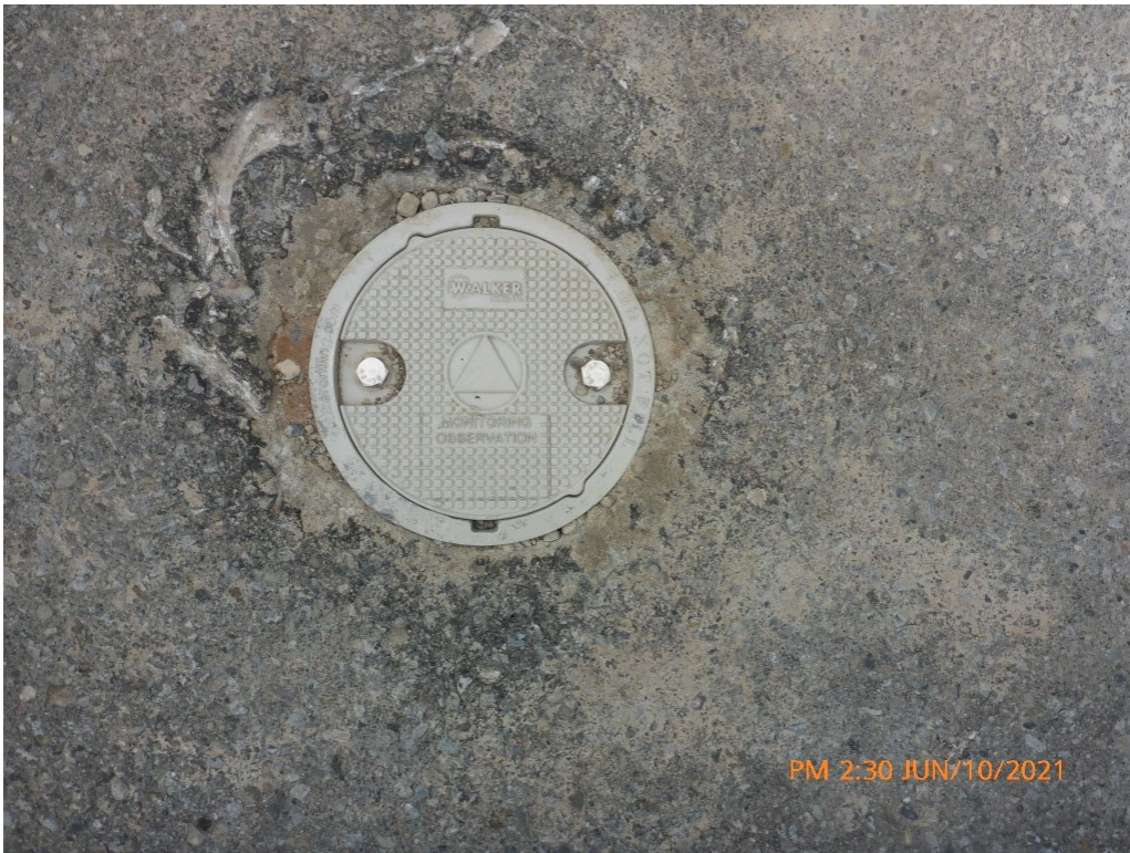
Approaches - Wearing Surface - Monitoring Well - West Approach - Photo 6
