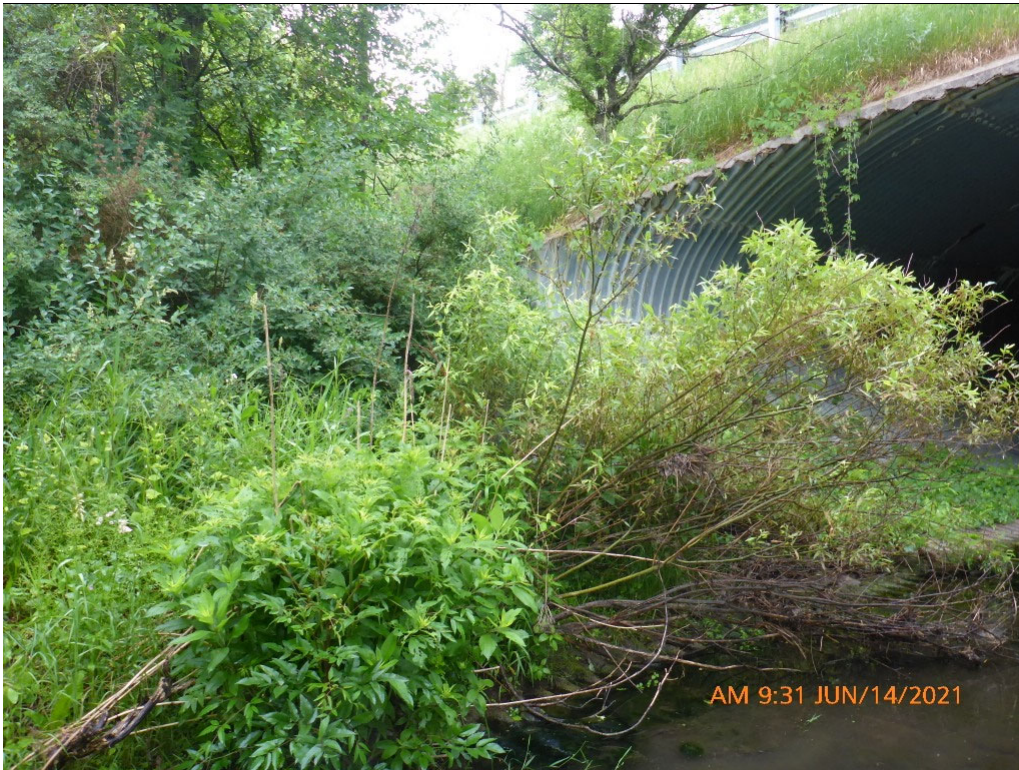
Embankments and Streams - Embankments - Vegetation Overgrowing Culvert at West - Photo 37
