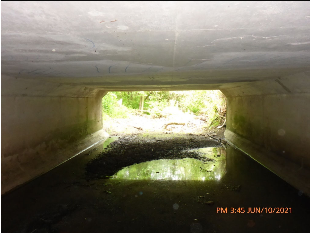
Looking East through Barrel at Midspan - Photo 7
