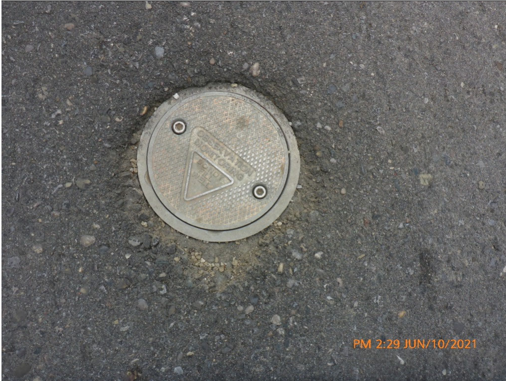
Approaches - Wearing Surface - Monitoring Well - East Approach - Photo 5
