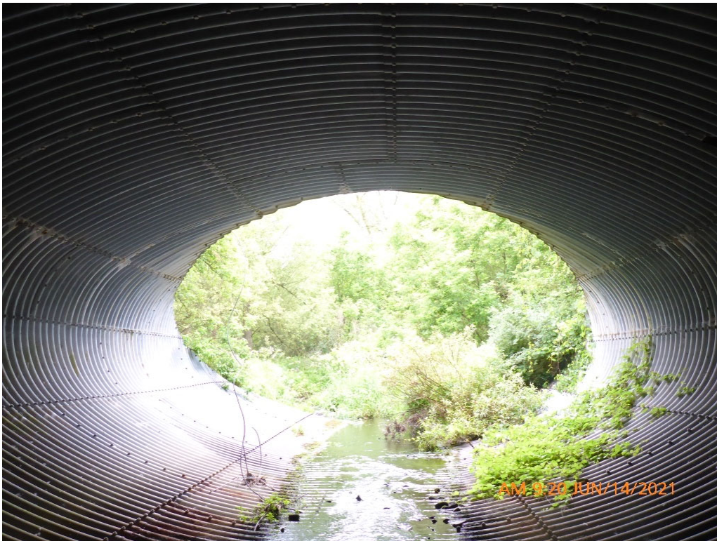
Looking West through Barrel at Midspan - Photo 10
