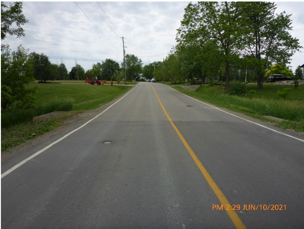
Looking West at Bridge - Photo 2
