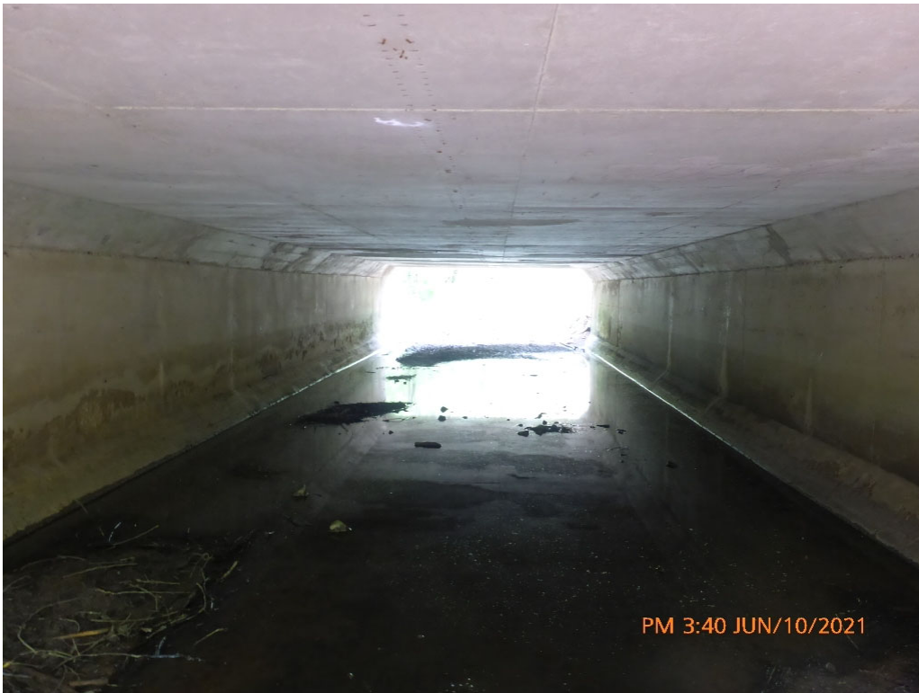
Looking East through Barrel from End - Photo 6
