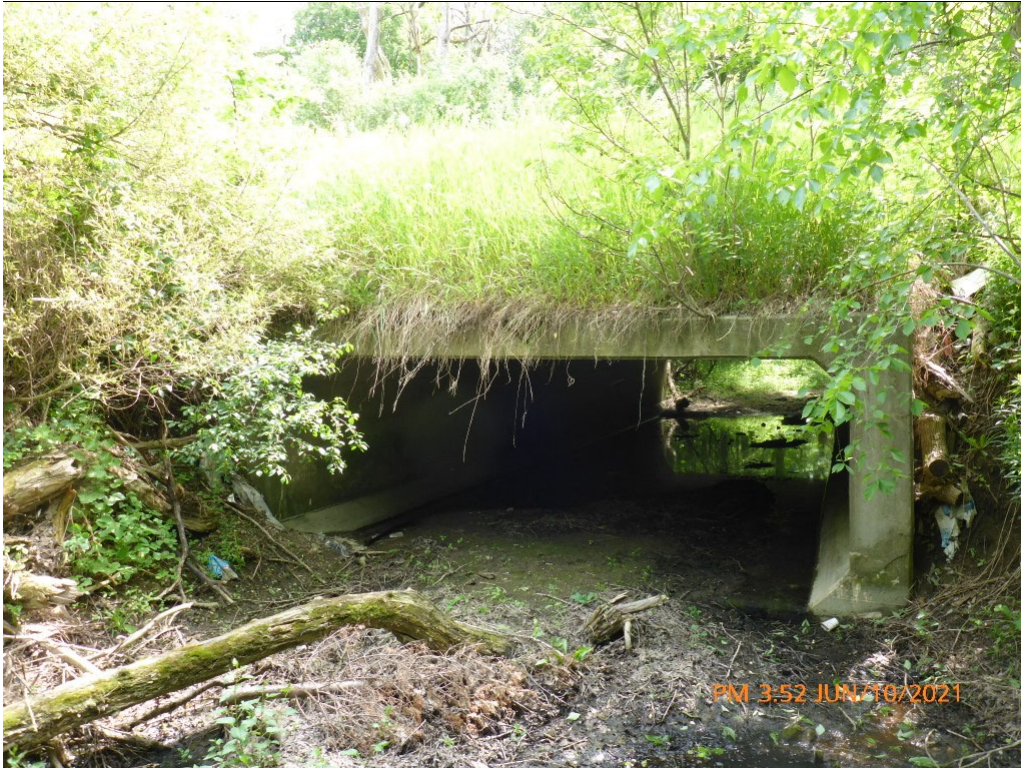
East Elevation - Photo 3
