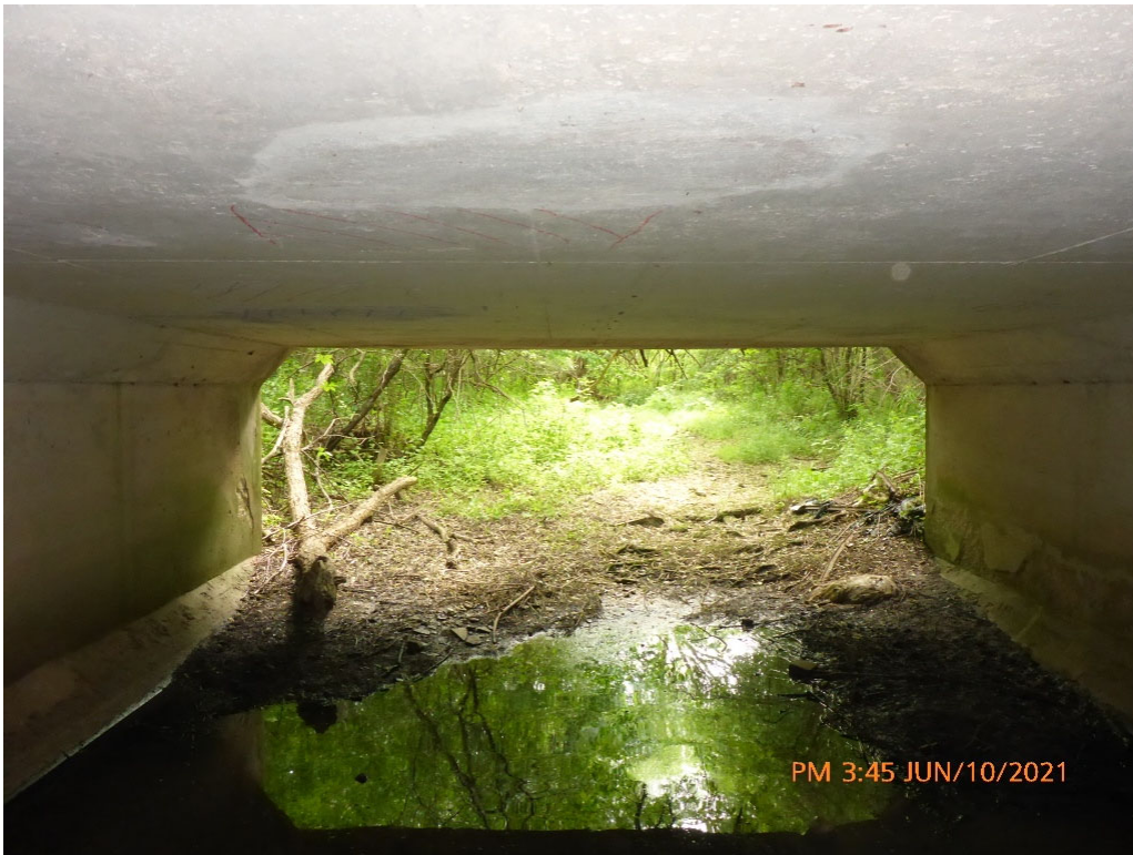
Looking West through Barrel at Midspan - Photo 8
