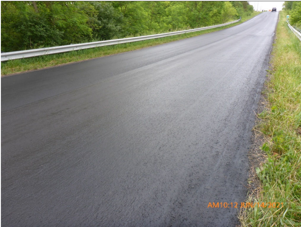
Approaches - Wearing Surface - New Surface Treatment over Structure - Photo 5
