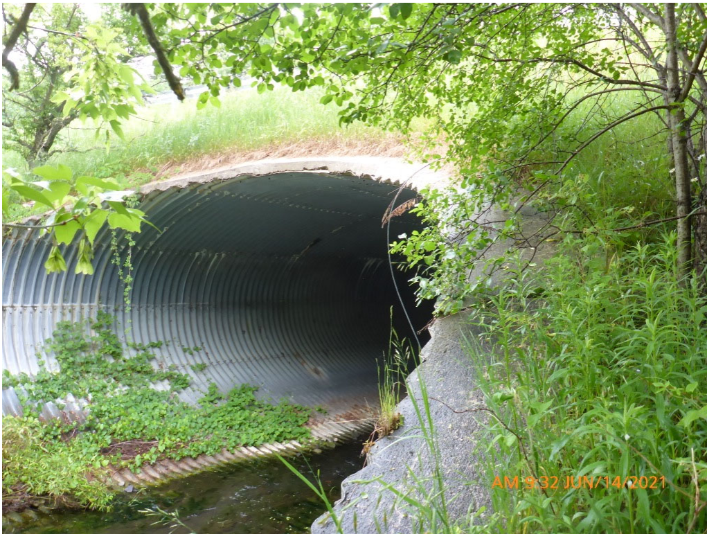
Culverts - Inlet Components - Typical Stiffener - Photo 24
