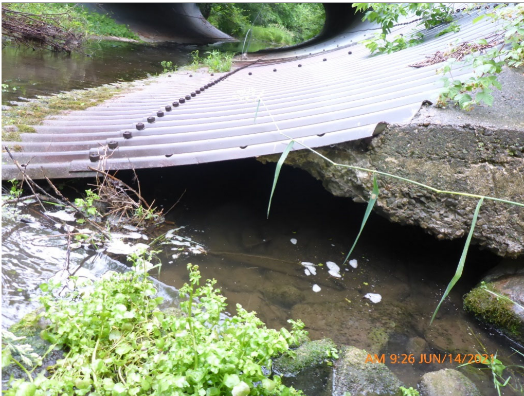
Embankments and Streams - Streams_Waterways - Severe Undermining of Barrel at West - Photo 38
