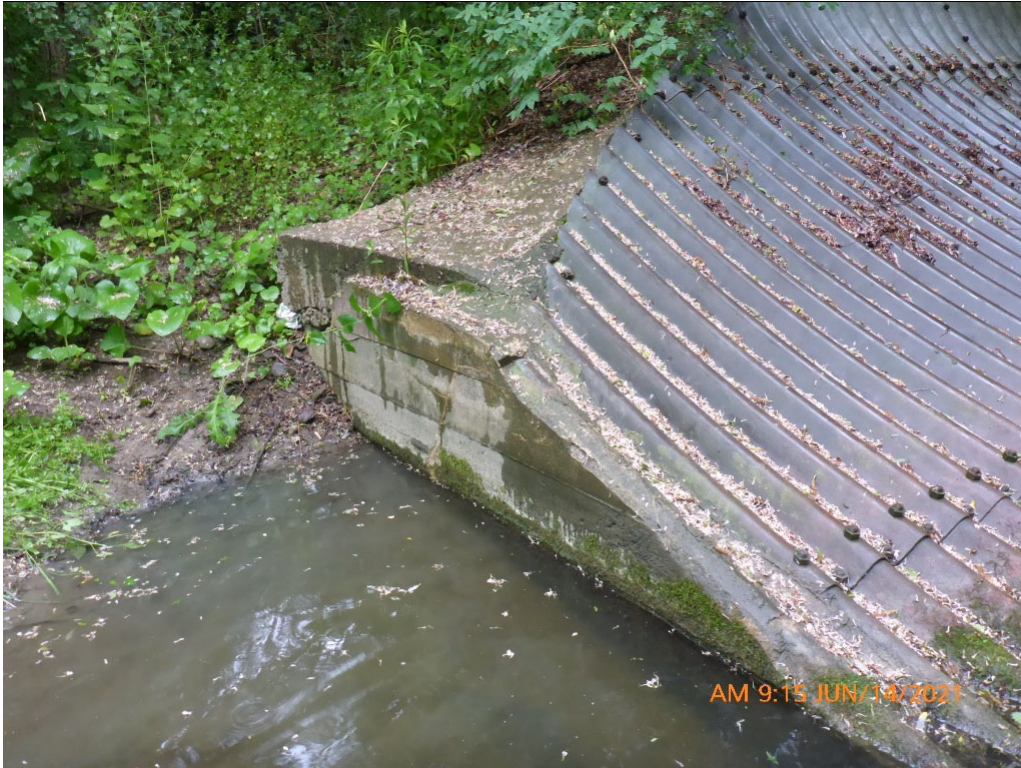
Culverts - Outlet Components - Typical Cut-off Wall - Photo 31
