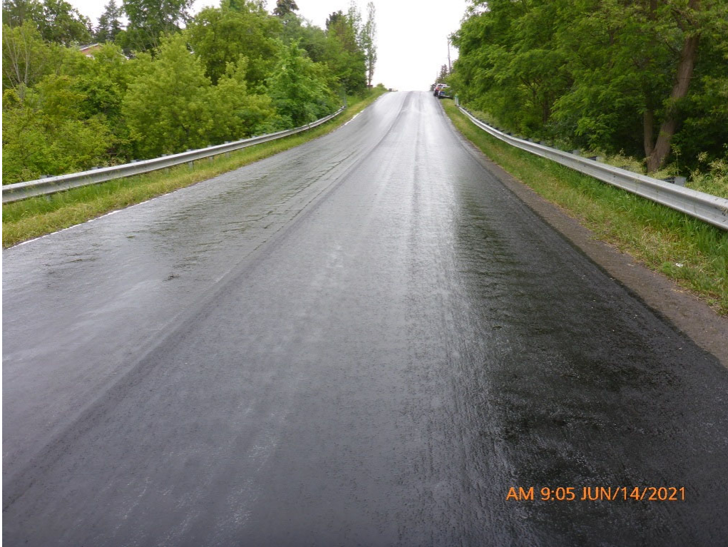
Looking North at Roadway over Culvert - Photo 1
