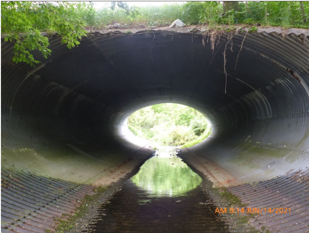
Looking West through Barrel from End - Photo 11
