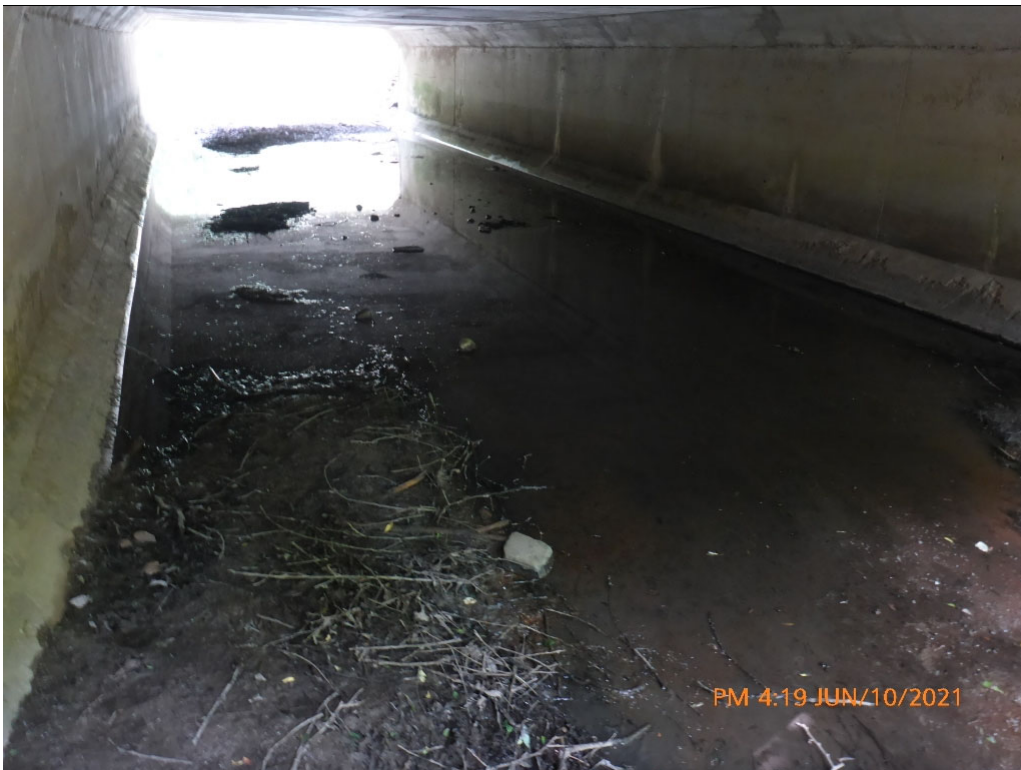
Embankments and Streams - Streams_Waterways - Watercourse through Structure - Photo 22
