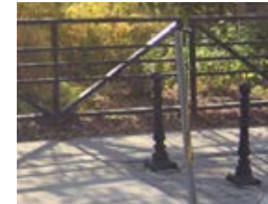
Example of existing bollards
