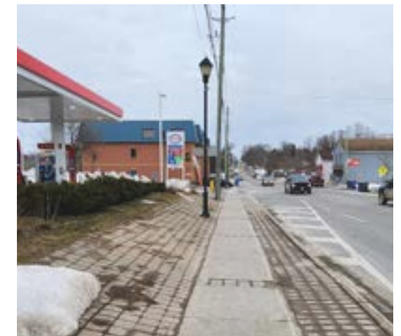
Example of existing sidewalk along Airport Road
