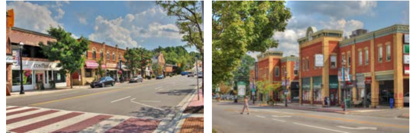
The above images illustrate the consistency in built form and setbacks within the commercial core of Bolton.
