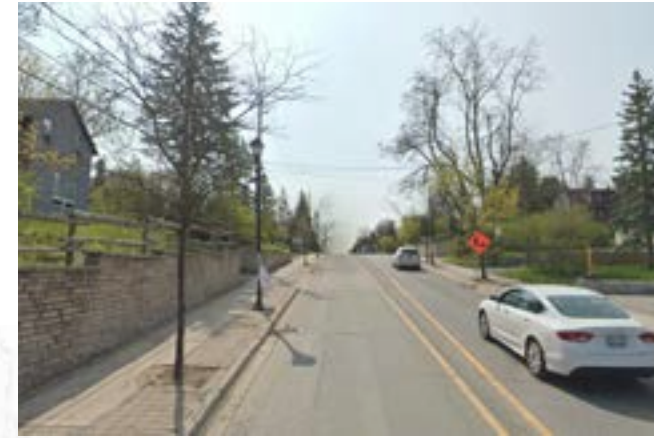
An example of retaining wall conflict within the Airport Road right of way
