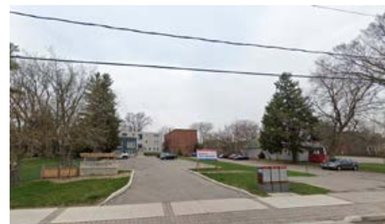
Existing conditions at 16069 and 16061 Airport Road
