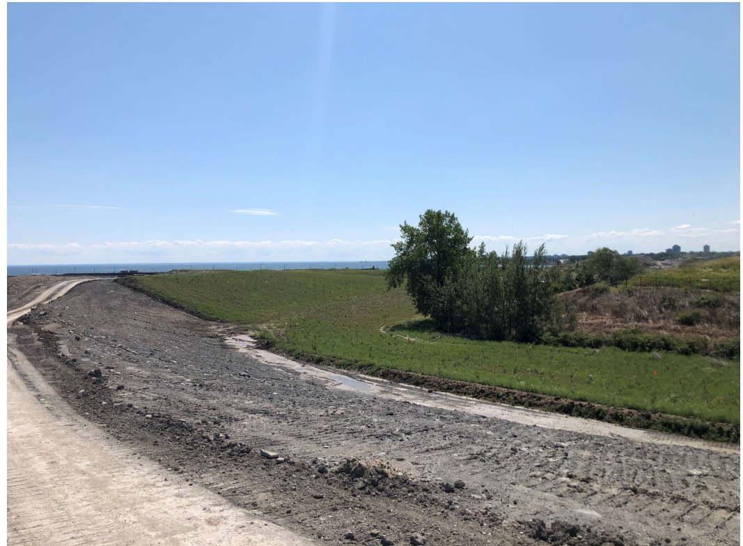
JTLCA Restoration in Progress
