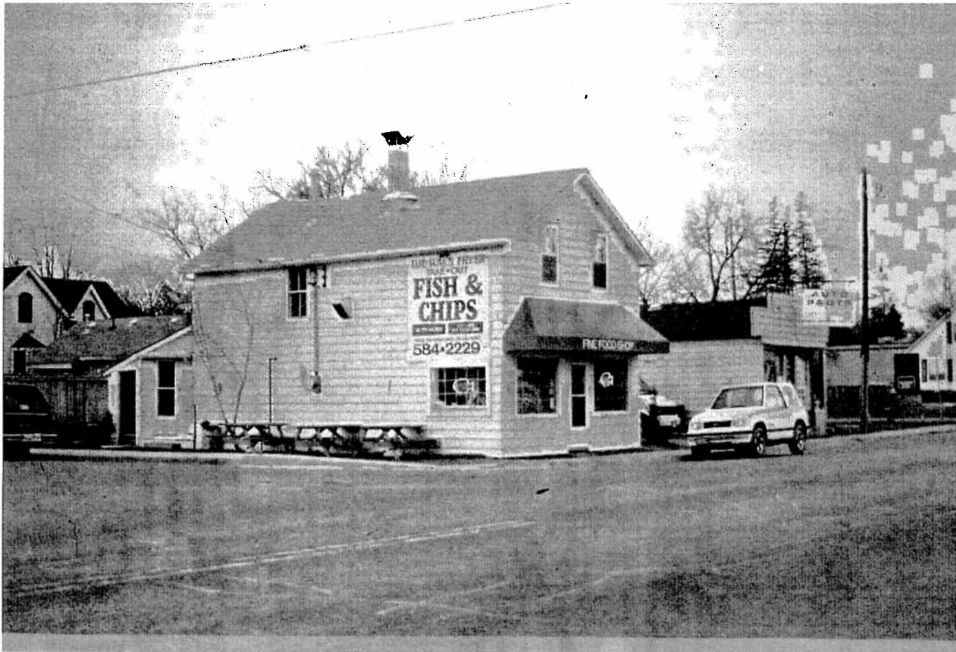
Figure 22 - This simple approach to the reuse of an existing building, although not restoration, has many positive features, a simple well proportioned canopy, sidewalk oriented entry and display windows and picnic tables. The scale and feel of the building is maintained.
