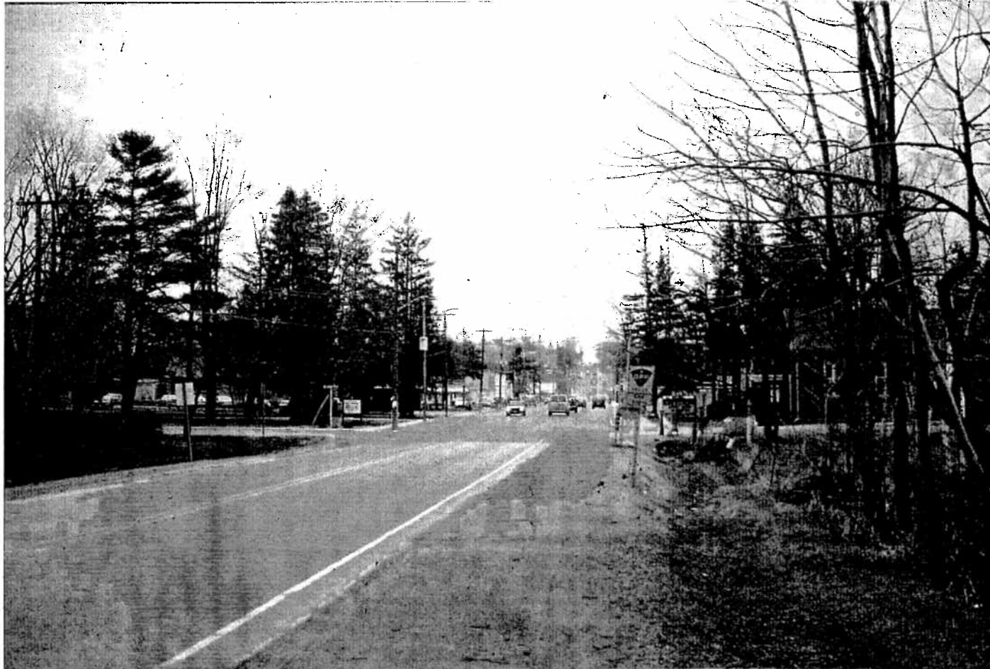
Figure 1 - Caledon East core area looking south
