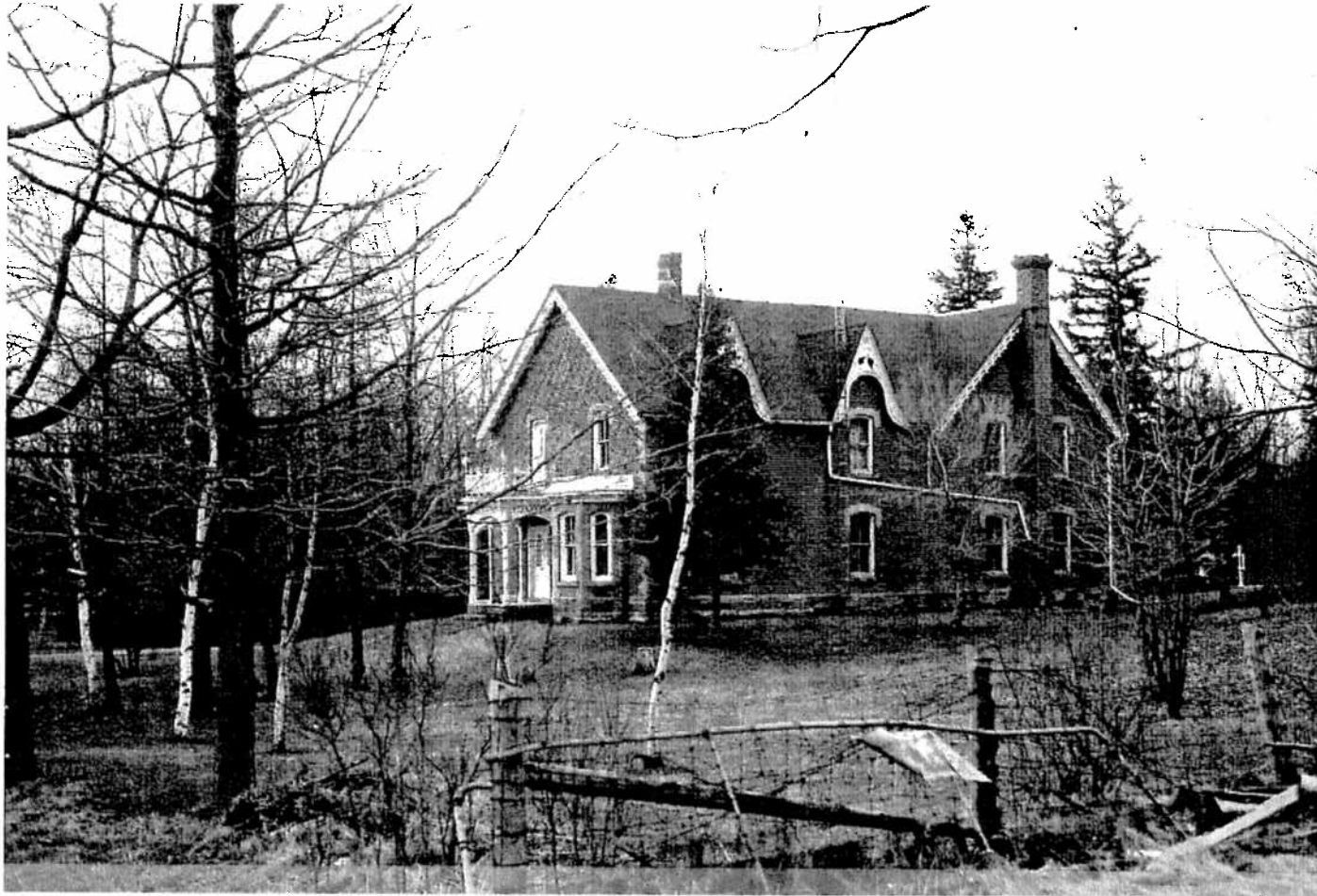
Figure 40 - Part 6. This fine Victorian house in a park-like setting is an aesthetically pleasing and picturesque welcome to the village from the north.
