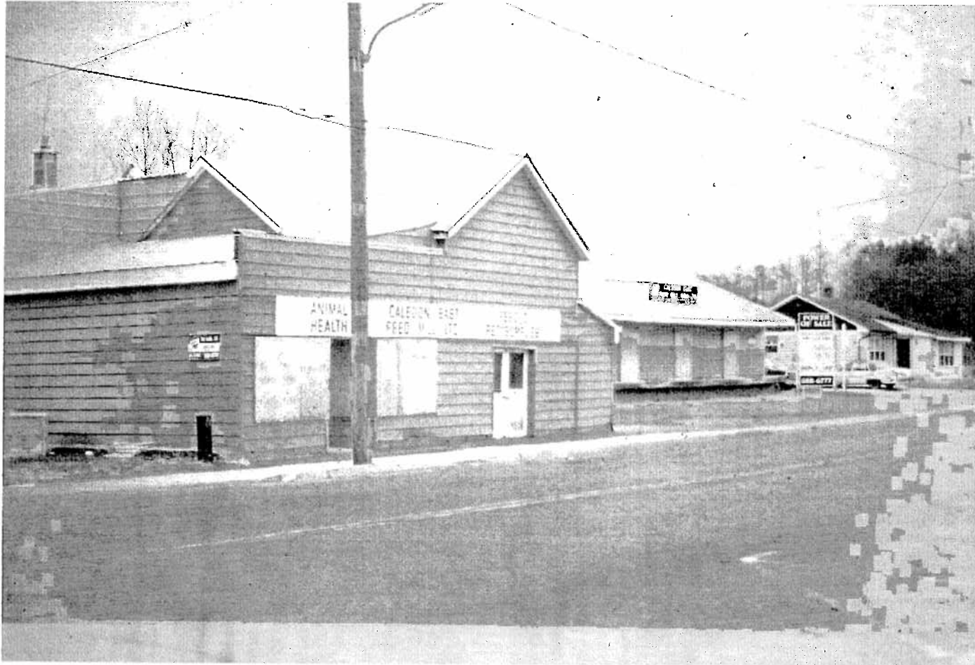
Figure 49 - This old feed mill site is the gateway to the core. A carefully planned development here could define the core edge, reinforce the core building patterns and establish the style and pedestrian orientation desired.
