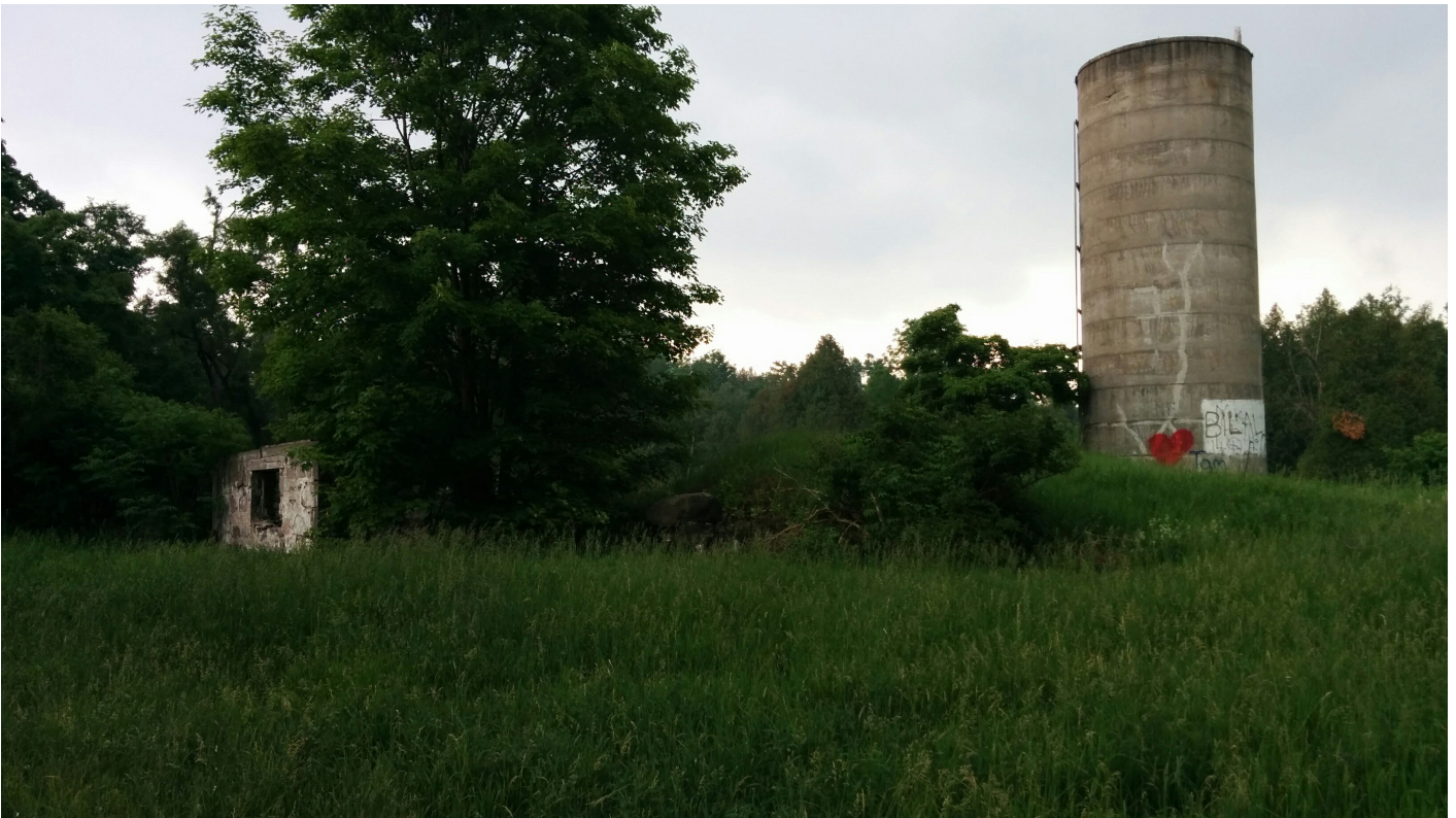
Figure 10: Photo of Existing Condition
