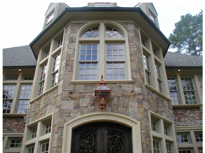
Figure 73: Example of window surrounds including lintels and sills in harmony with the architectural style
