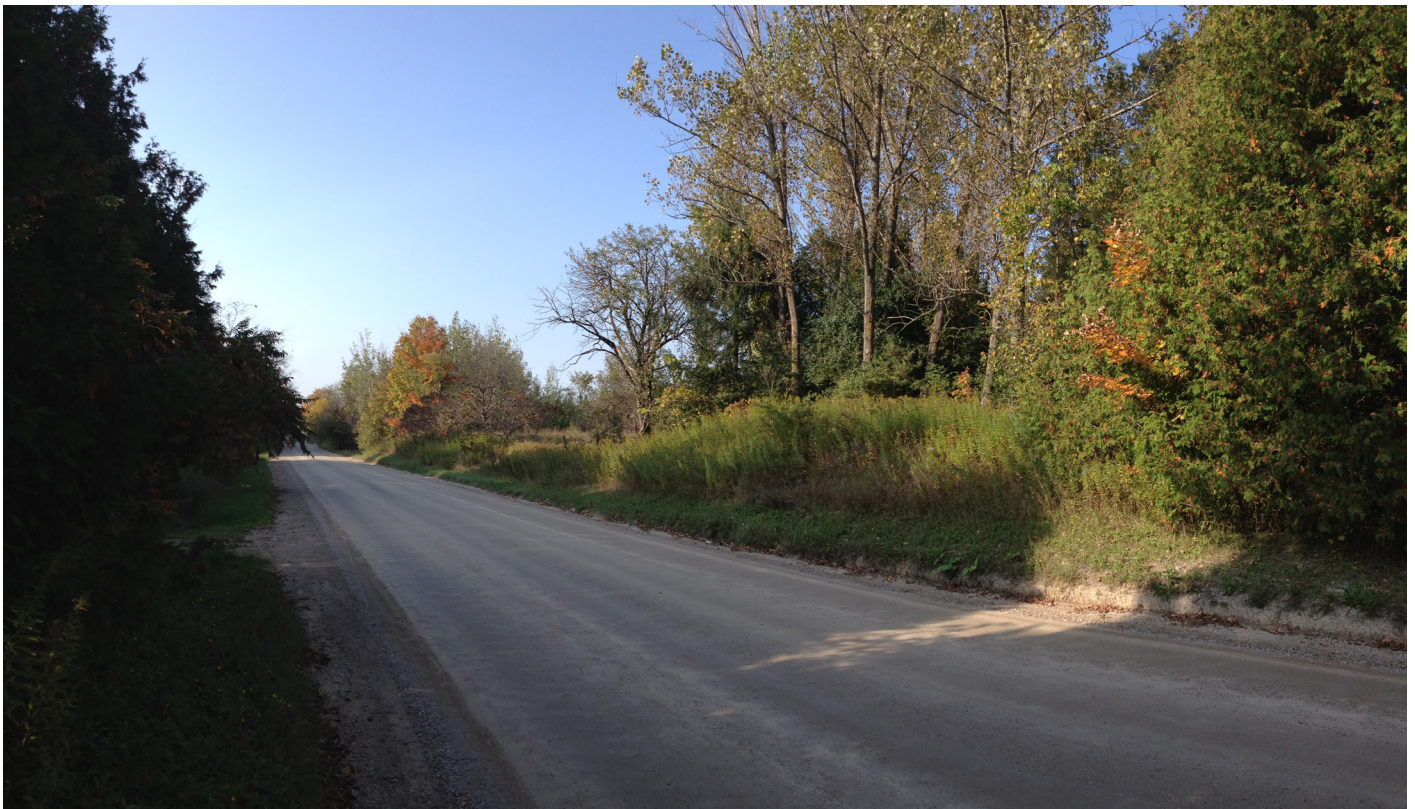
Figure 05: Photo of Existing Condition
