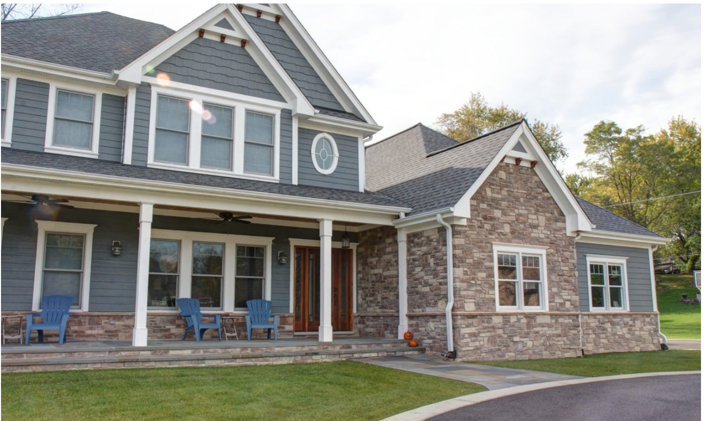
Figure 71: Example of a combination of fieldstone and wooden siding materials
