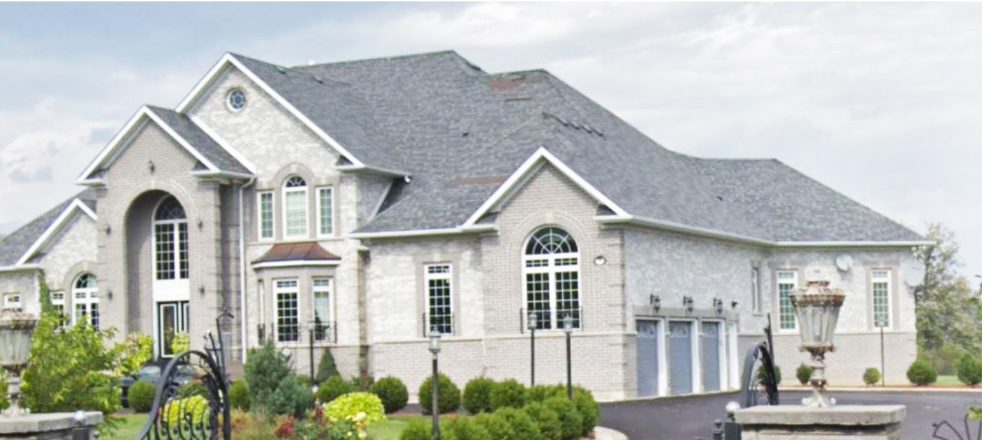
Figure 76: Example of side facing garage with enhanced facade treatment facing the street
