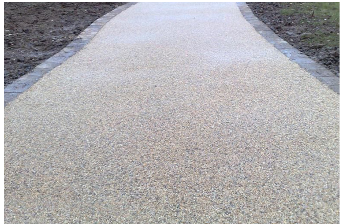
Figure 29: Tar and Chip Driveway
