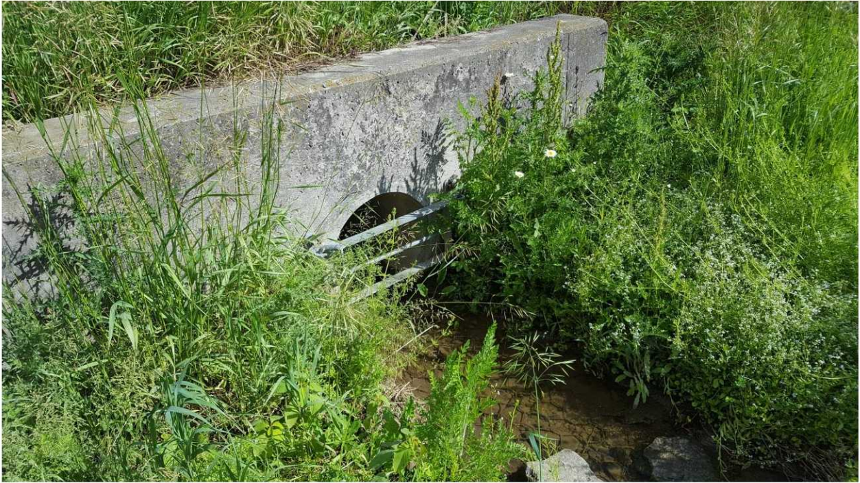
Photo 5 – Outlet of 66 cm diameter culvert near east end of northwest field.
