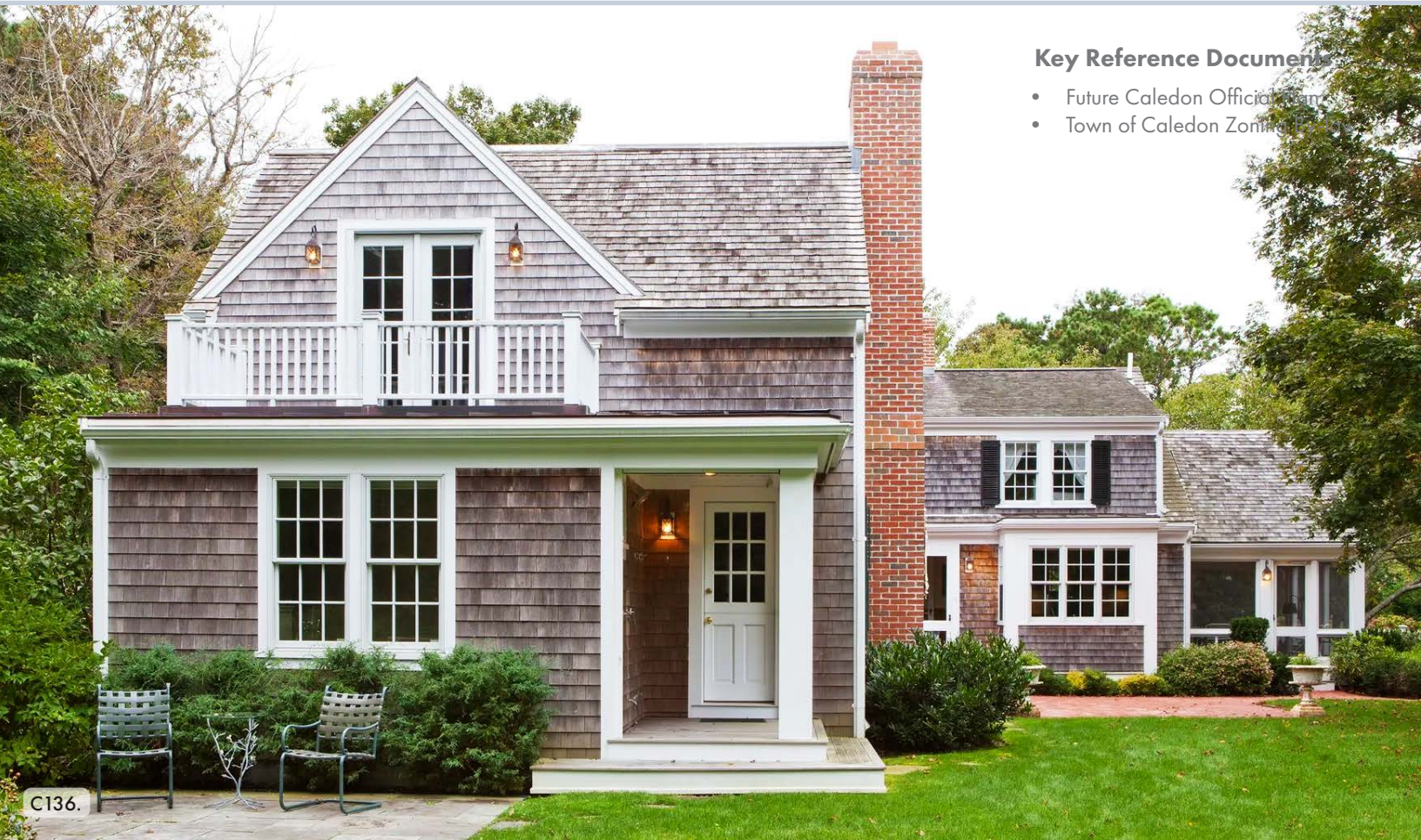
C136. A single family dwelling with an ARU addition, thoughtfully integrated to preserve the home's original character through the use of similar materials, colours, and proportions.
