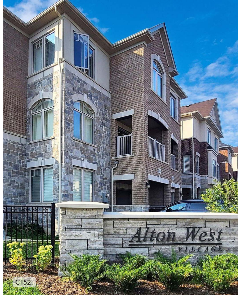
C152. A gateway lot landscape treatment that serves as a landmark within the community.
