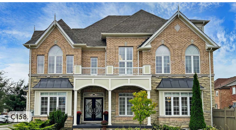
C157. Diagram example of a corner dwelling. C158. Elevation with wall plane changes, projecting bays, and gable features.
