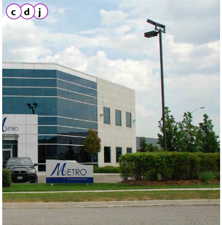
Example of downcast solar PV lighting (Vaughan, ON).
