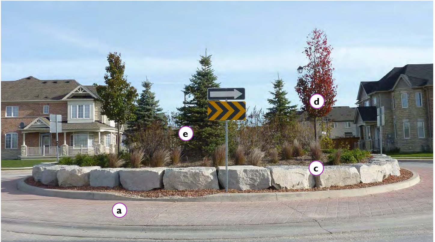
The roundabout in Mayfield West is designed with hard and soft landscape elements.
