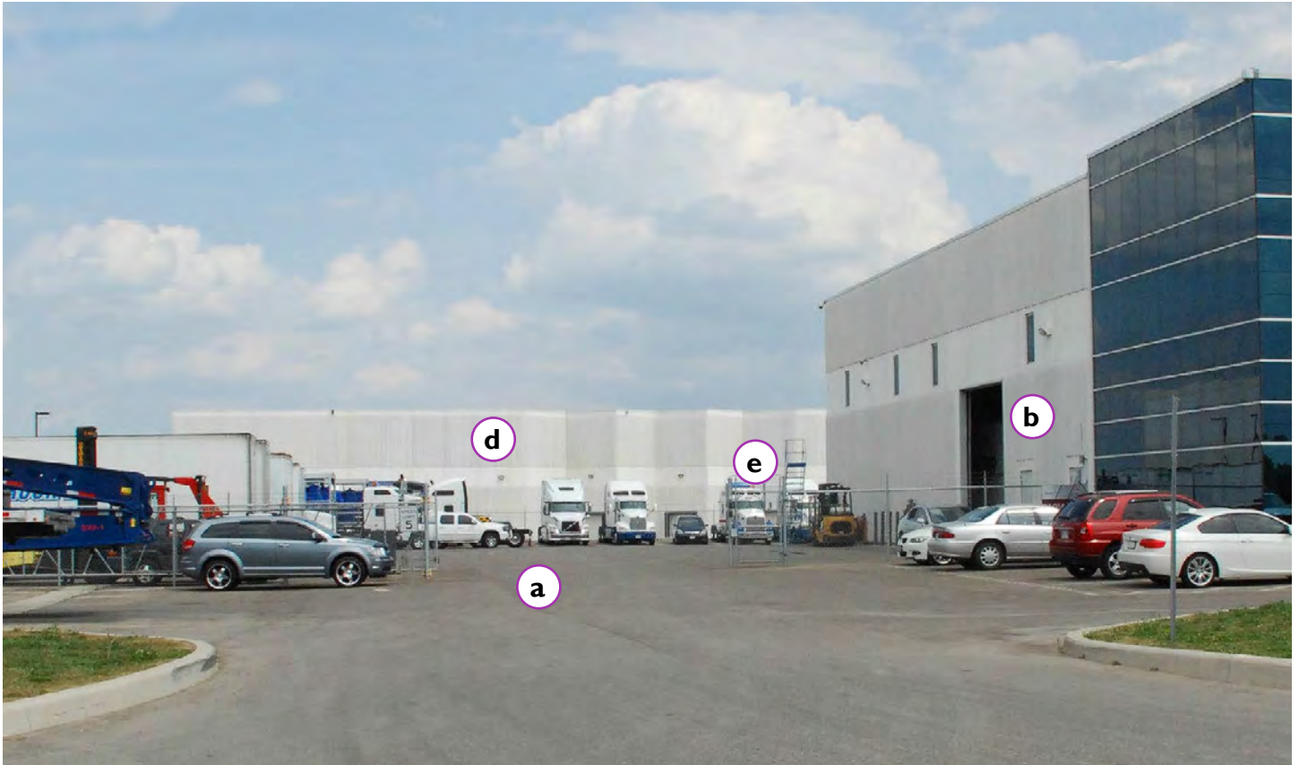
An example of an outdoor loading area that is located at the rear of the building, away from the main street.
