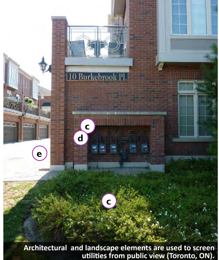
Locate utilities away from the front façades, in the rear of buildings and coordinated with parking facilities.
