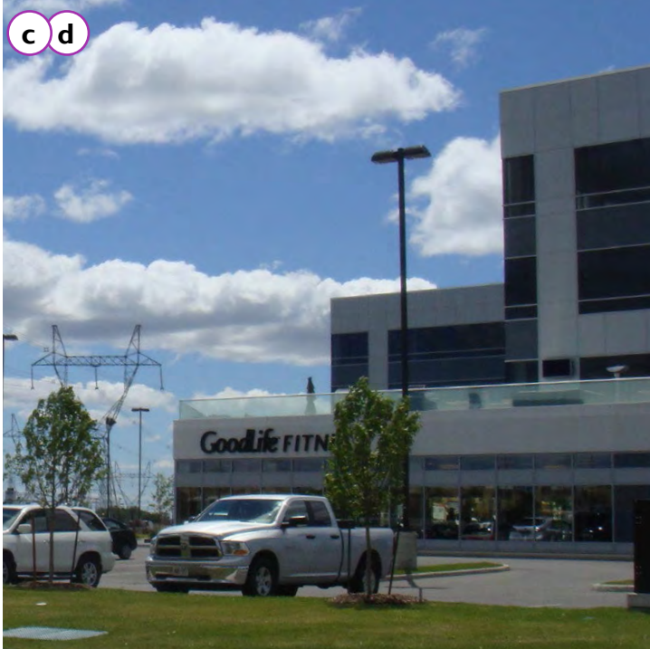
Site lighting is downcast at the Adidas Headquarters in Vaughan.
