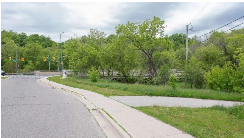
Picture 23. Sidewalk abutting roadway (Caledon, ON)
