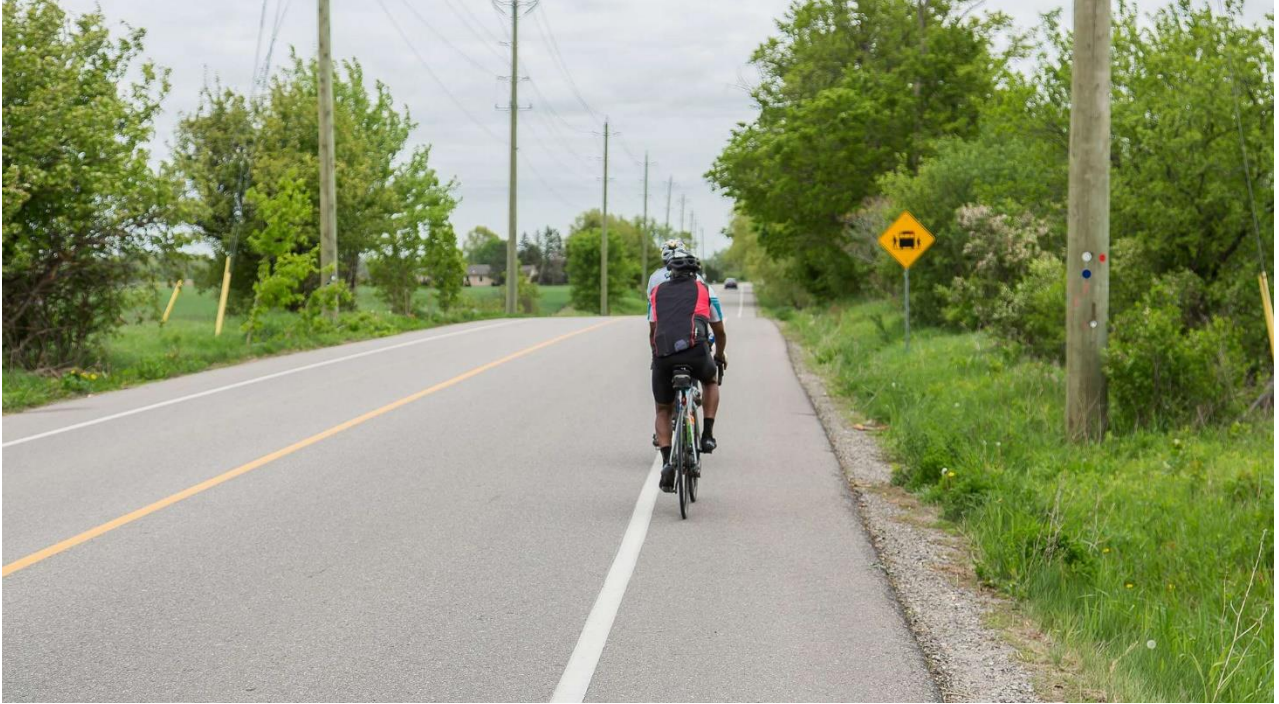
Paved shoulder (Caledon, ON)
