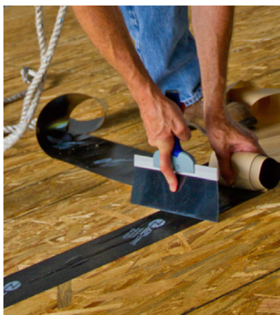
Basic secondary water barrier: Roof deck taping to seal seams between sheathing panels
