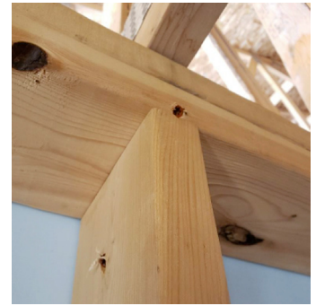
Example installation of truss screws to enhance connection between top plate to truss, and stud to top plate.
